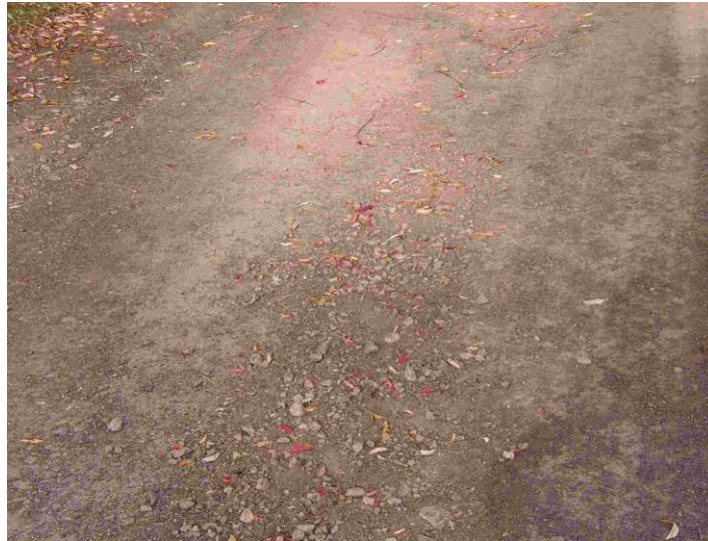
Fig. 1: Detailed view of the modified road cover.
