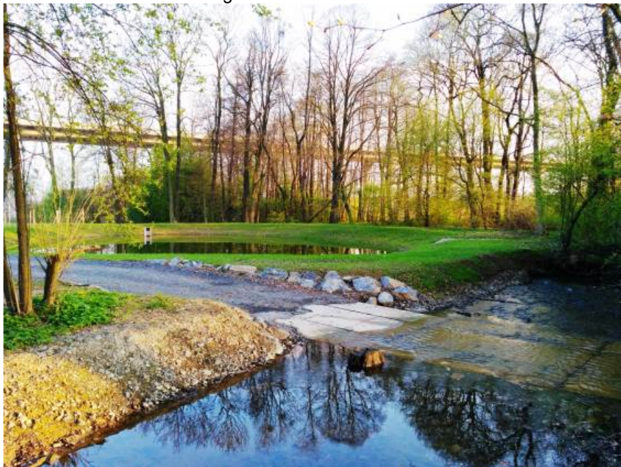
Fig. 2: Water bio-centre in Bělotín
