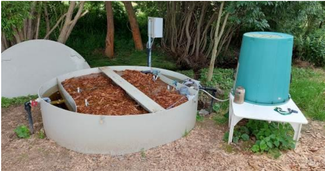
Fig. 3: View of the internal layout of the combined bioreactor including the woodchip charge
