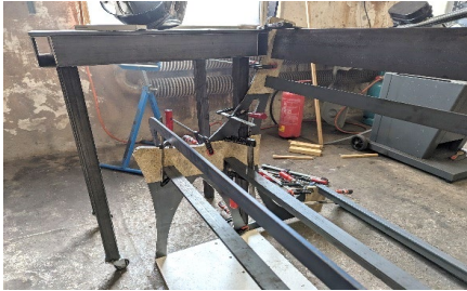
6: Creation of the structure before removing the templates
