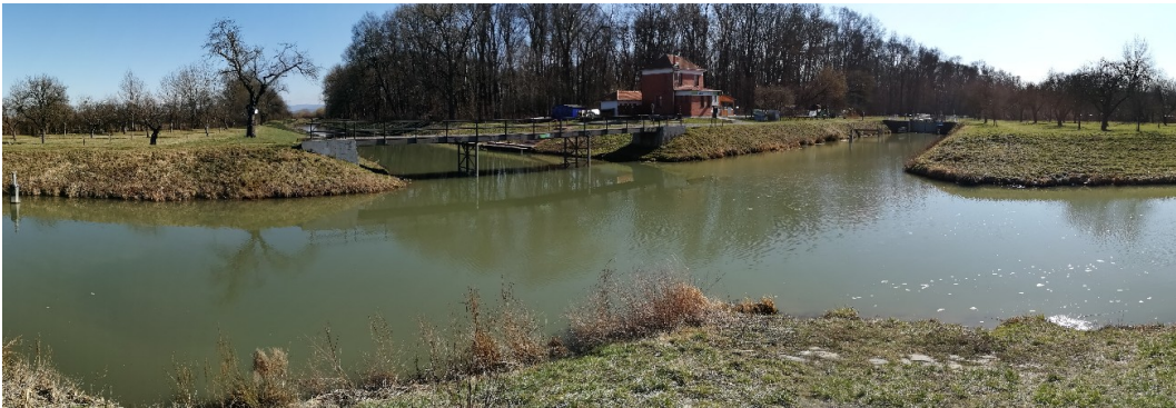
Fig. 3: An example of a functional unit of water management systems with a flood control function, irrigation function and transport waterway (Pomoraví, Baťa Canal, Czech Republic), in which the social function (support and use within tourism) has gained importance.
