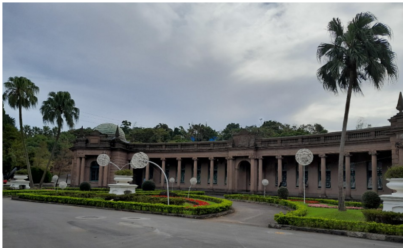
Fig. 1: View of the historic pumping station of the water utility complex, which serves as a museum, part of an educational and entertainment water park, and as a backdrop for cultural and social events (Taipei, Taiwan).
