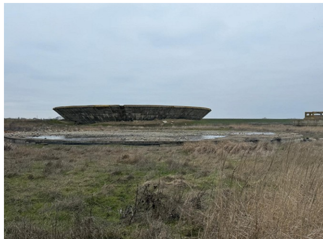
Fig. 4: The ruins of a vessel from the water cooling plant at the Călărași Steel Plant
