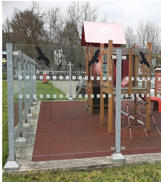
Fig. 3: Glass screens at the playground prevent flying objects from passing through
